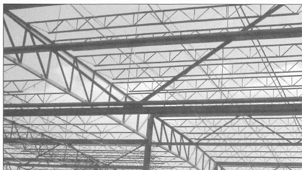
Fig. 3–11. Metal bar joist trusses
