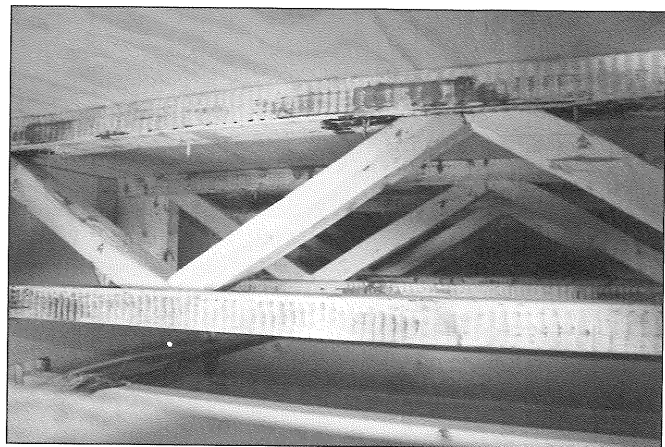
Fig. 2-103. A finger joint truss was used in this modular home to support the second floor. Courtesy of Kevin Gallagher.
