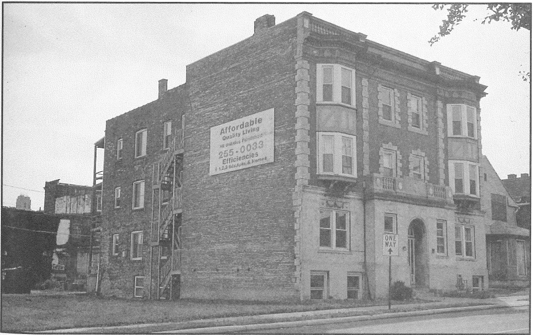
An ordinary constructed (exterior walls of brick or block) Apartment Building. Credit Coleman
