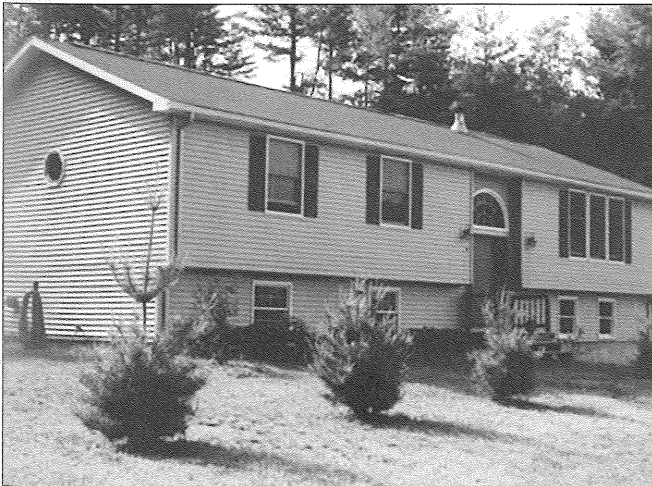
Fig. 2-88. This home is an example of modular construction. Courtesy of Kevin Gallagher.
